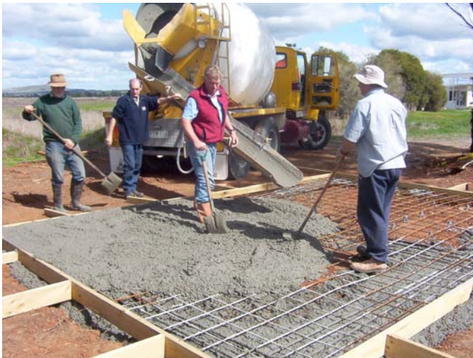
Pouring the slab for the town shelter
