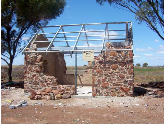
Shelter with prefabricated roof in place.
