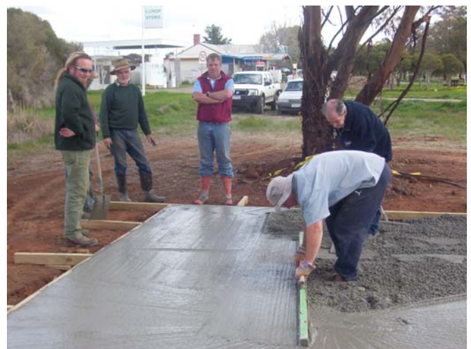
CCAG members pour the 16 cubic metres of foundations and slab.
