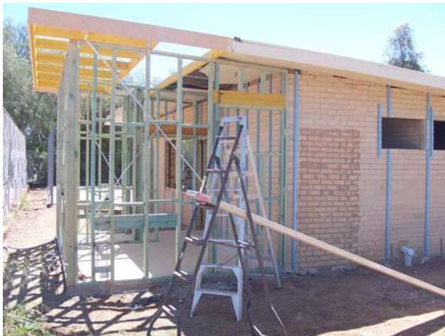
Framework for the upgrade to the toilet facilities takes shape
